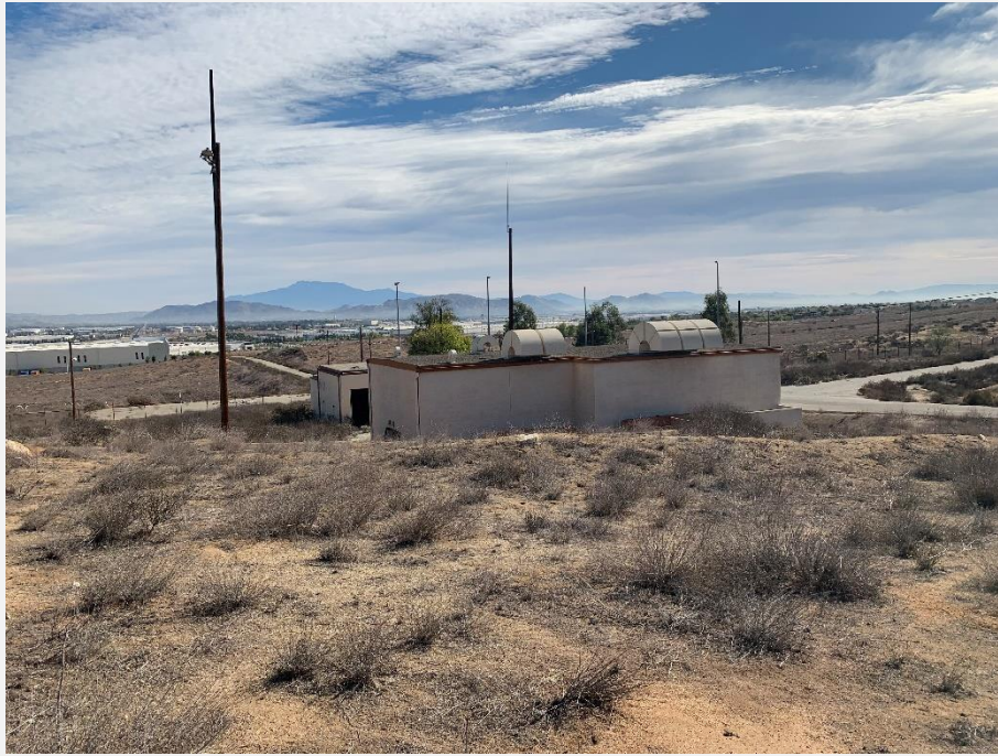
Photograph 25. Photograph taken inside the fenced retired AFB facilities area of existing structures located at the eastern end of Arclight Drive. Photograph taken facing east/southeast.
