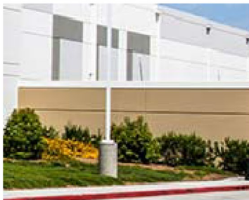
TILT-UP CONCRETE SCREEN
