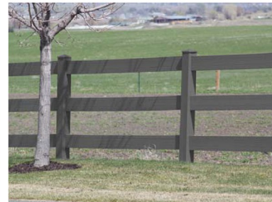
SPLIT-RAIL FENCING ALONG BARTON STREET MULTI-PURPOSE TRAIL & TRAILHEAD LOCATIONS- COMPOSITE, MATTE FINISH
