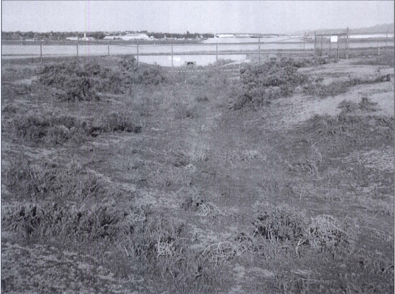
Figure 1. Northwestern portion of the flood control channel where it drains from a concrete pipe culvert located along the south side of a taxiway on March ARB (view to the north-northwest). From here, it drains southeasterly across the property and into a modern, concrete pipe culvert.
