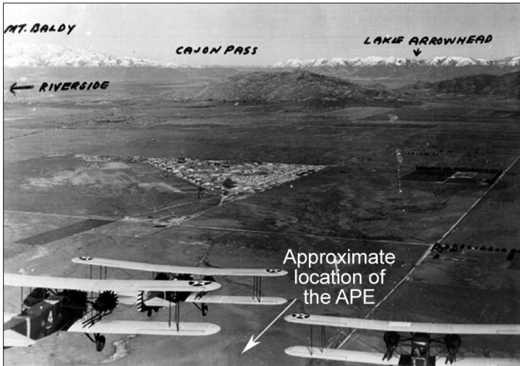
Figure 8. Aerial photograph of March Field and the APE location in the 1930s. (Source: March ARB 2010)
