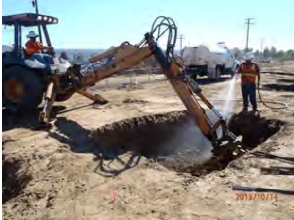
Soil conditioning and compacting excavation
