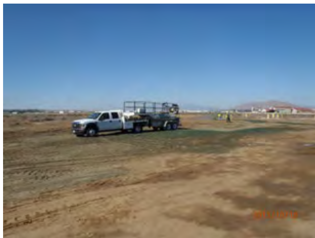
Hydro Seeding the excavation area, looking NW
