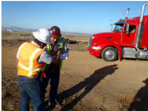
Signing Manifest for trucks hauling to Soil Safe of Ca. TPST in Adelanto Ca.
