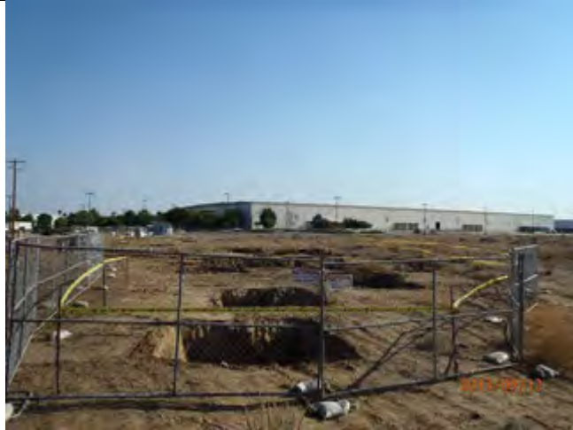
From NE corner of site looking South over secured excavation areas.
