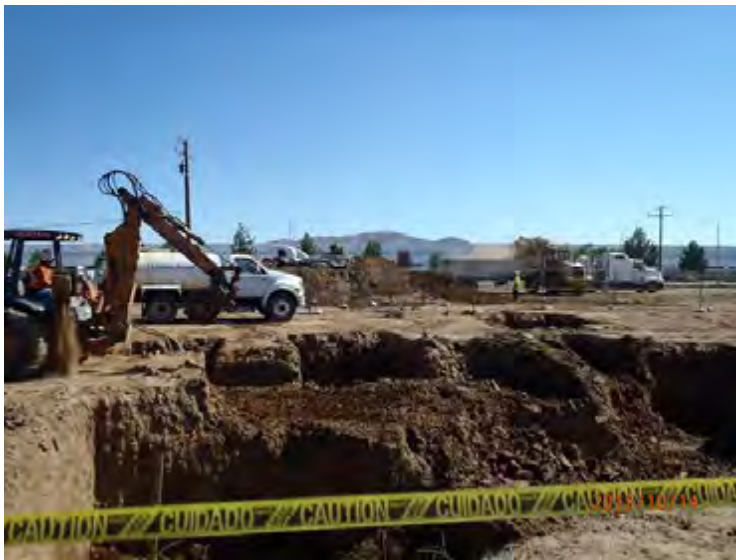
Loading out soil, dust control and excavation compaction and backfilling
