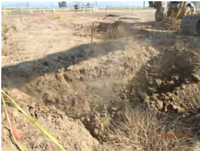
Slight gray staining observed. All discolored soil excavated out.
