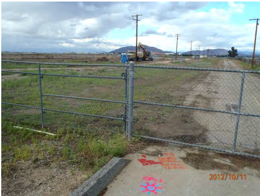
CalVeda Southern control pin location looking North onto the site from entrance gate
