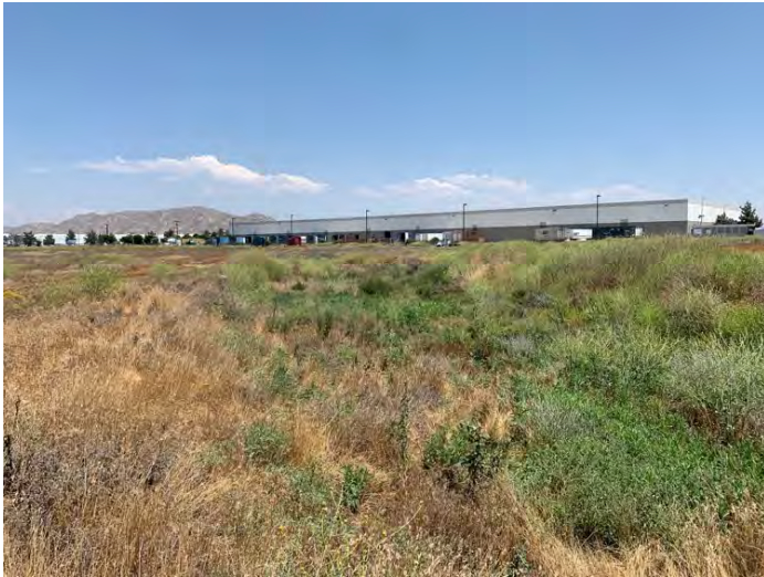
Photo 11. Downstream view of Non-Wetland Water (NWW)-1A/NWW-1, facing east. NWW-1A/NWW-1 begins to show stronger indicators of an OHWM from this point. (33.876444, -117.248193).
