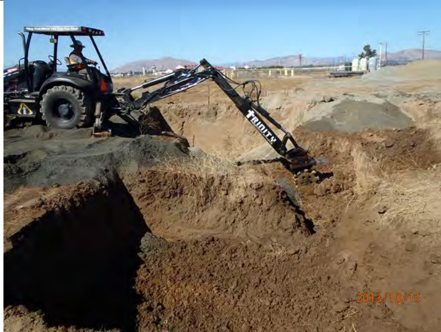
Soil conditioning and compacting excavation
