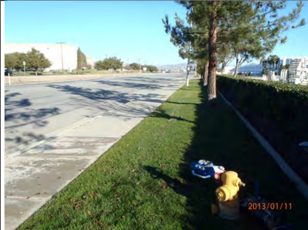
Water meter and backflow preventer ready for pickup by agencies, located about 300yd south of site
