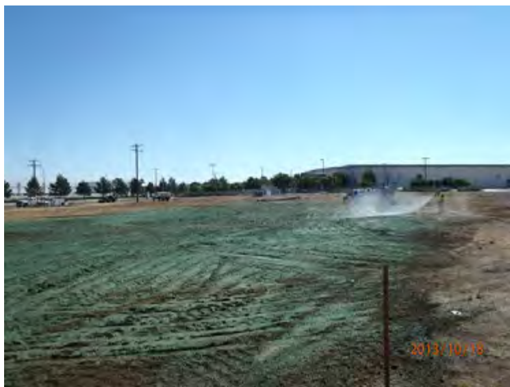
Hydro Seeding the excavation area, looking S from NW Corner
