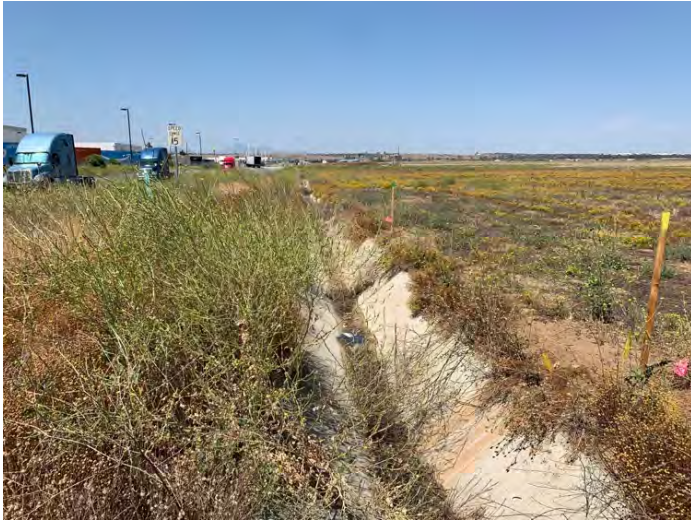
Photo 17. Overview of the middle segment of D-1. Photo taken facing west (33.876600, -117.245491).
