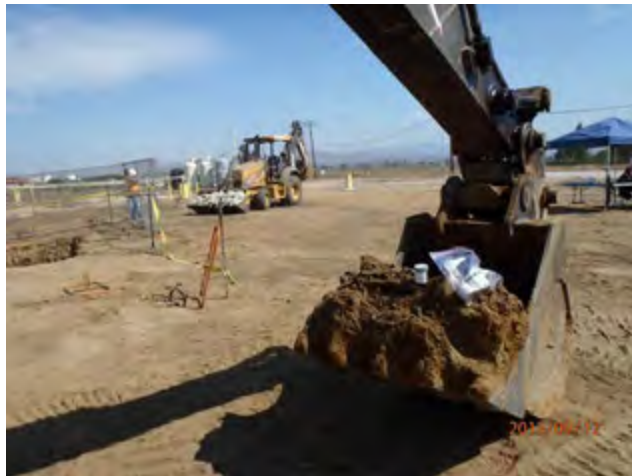
Obtaining confirmation samples and installing security fencing
