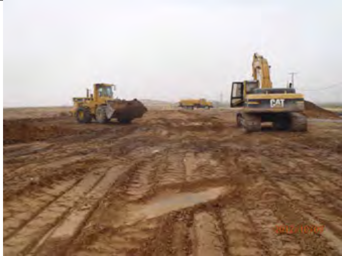
Excavating Site FT007 area, looking North from the South
