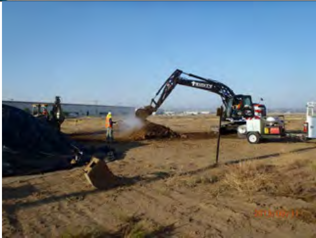
Dust control during excavation and stockpile work
