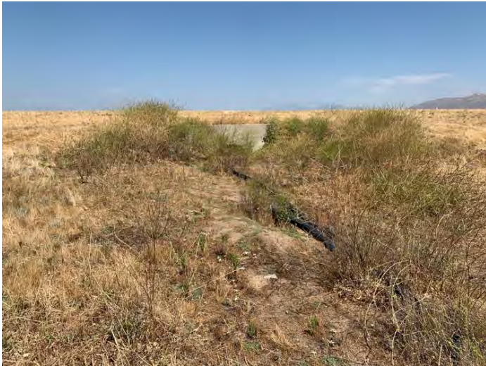
Photo 27. Overview of S-2, showing a culvert outlet. Photo taken facing north (33.878071, -117.249947).
