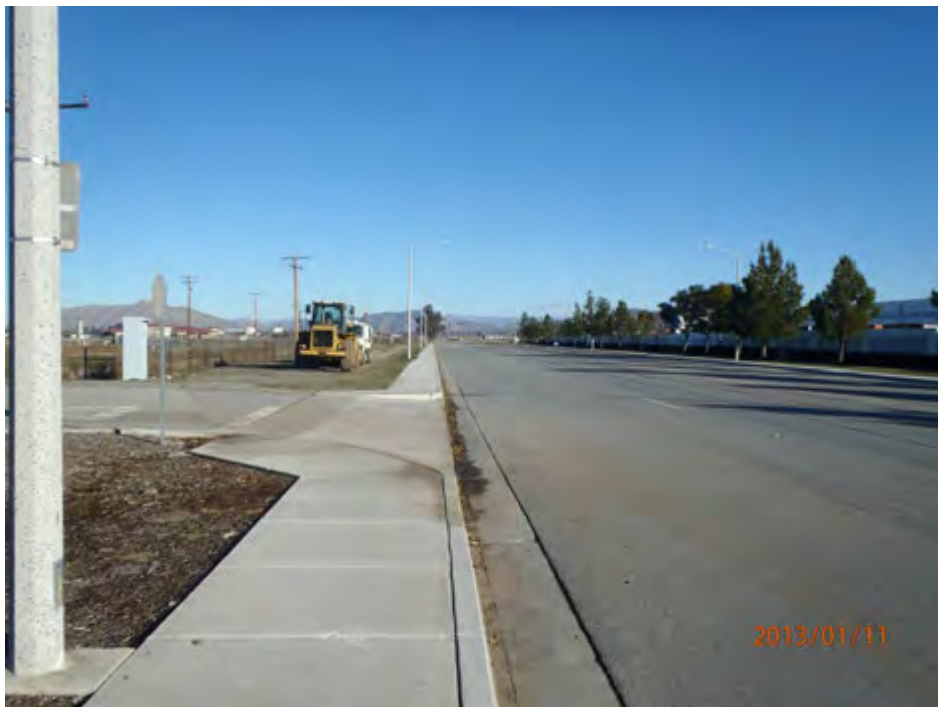
Street entrance cleaned, looking north
