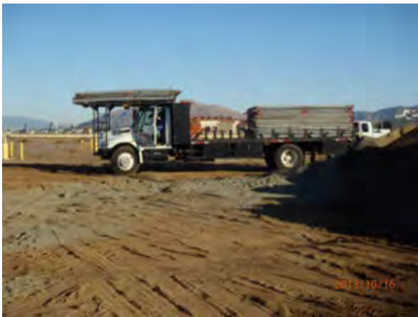
National Rent a Fence picking up the fence panels
