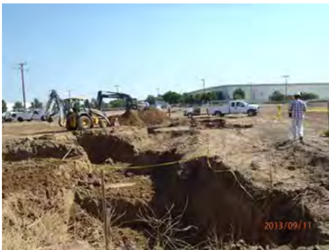
North side of deep excavation area looking South
