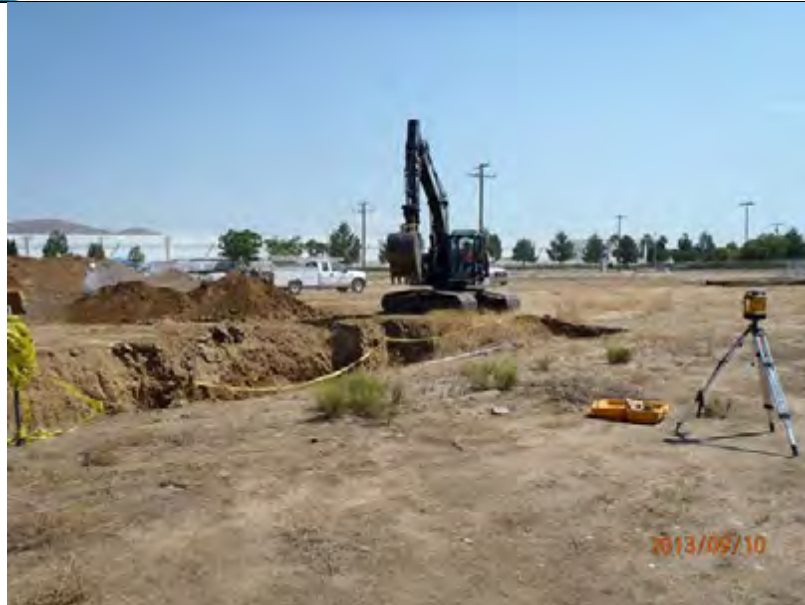
Excavating & stockpiling soil, using laser to verify depth of excavations
