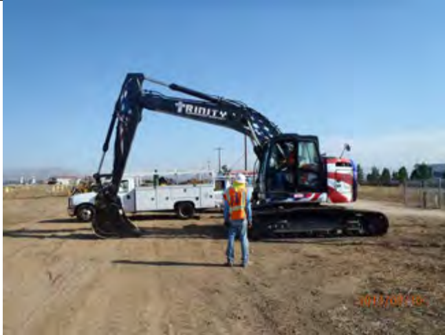
Inspecting new Excavator prior to use
