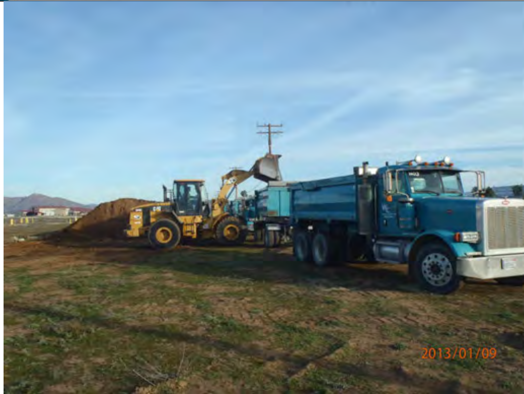
Loading truck out.
