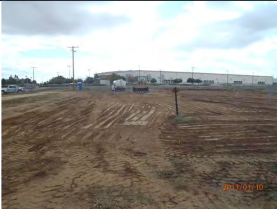
Stockpile loaded out and area cleaned up.
