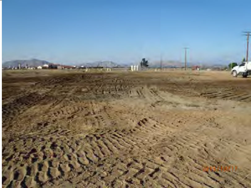
Backfill completed, looking North from SW corner
