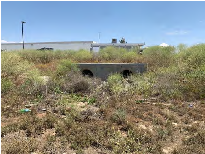
Photo 15. View of the on-site terminus for NWW-1A/NWW-1 at two culvert inlets (33.875766, -117.247498).
