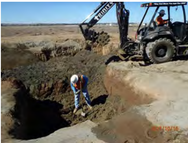
Soil conditioning and compacting excavation with Norcal performing soil compaction testing
