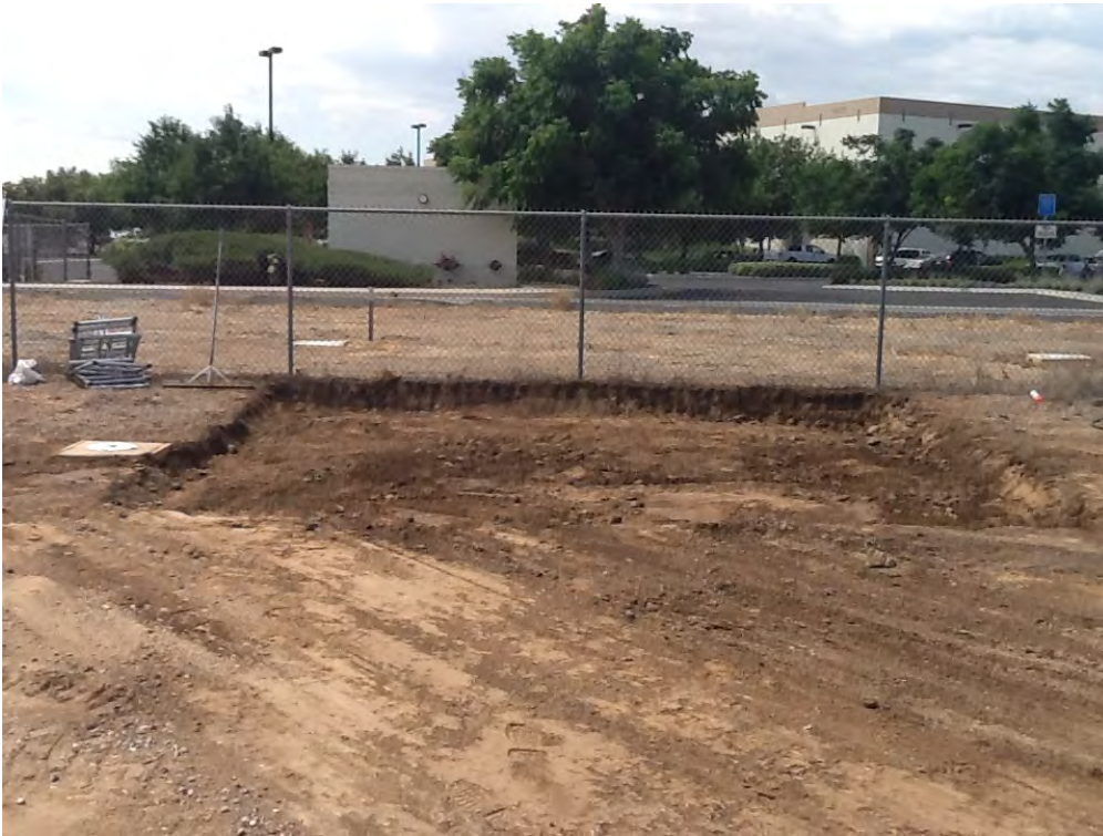
Soils were excavated to 6 inches below grade for the SVE pad.
