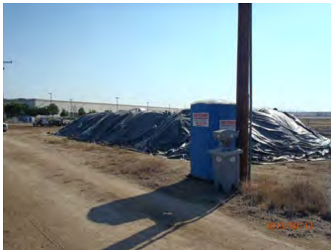
Looking SW at secured Stockpile
