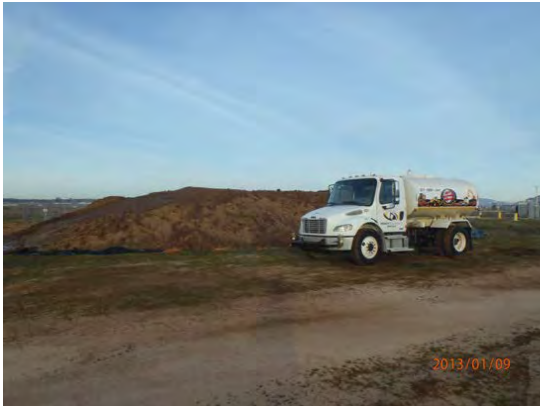
Wet down stockpile and haul routes
