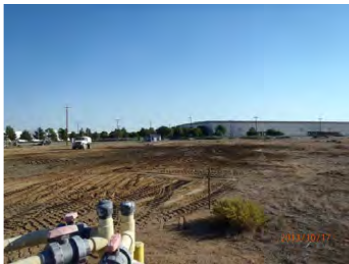
Backfill completed, looking South from NW corner
