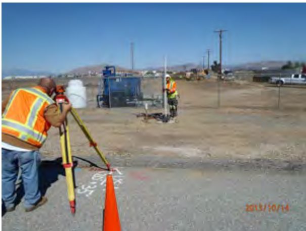
Surveyed in excavations perimeters, sample locations, and well locations
