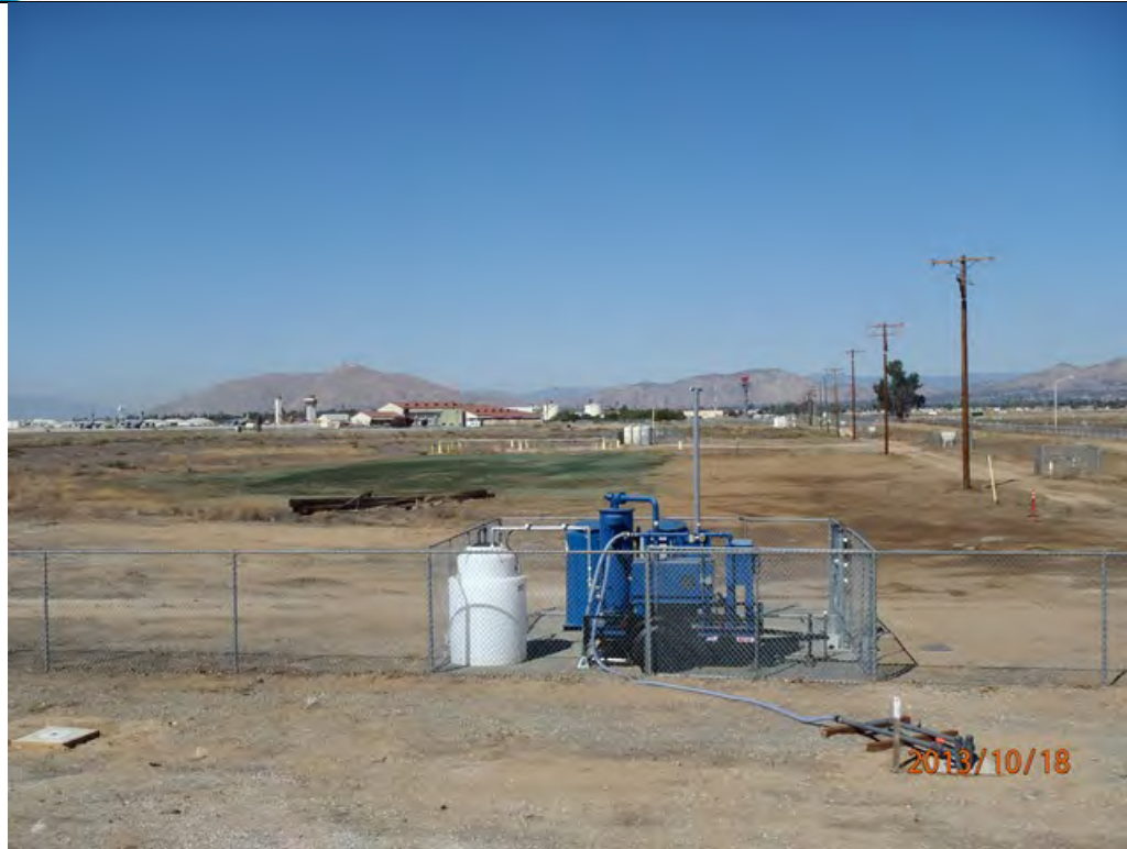
Hydro Seeding completed, Site cleaned and equipment demobed, Looking N.
