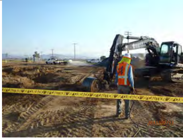
Excavating and site dust control
