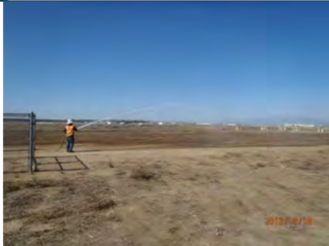
Preparing for Hydro Seeding, Looking NW
