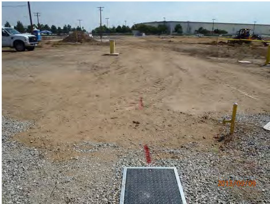
From NE corner of site showing alignment of new electrical line .
