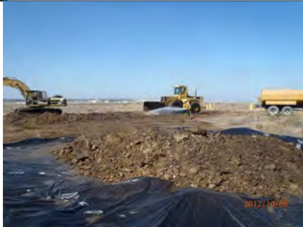
Excavating Site FT007 with dust control, looking NW from stockpile location
