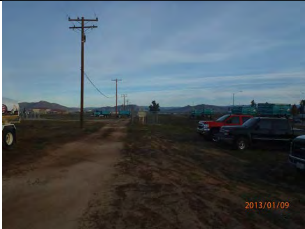
Directing truck traffic for one way loop safe truck and equipment movement
