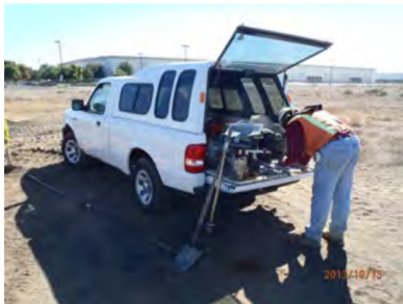
Norcal performing soil compaction testing
