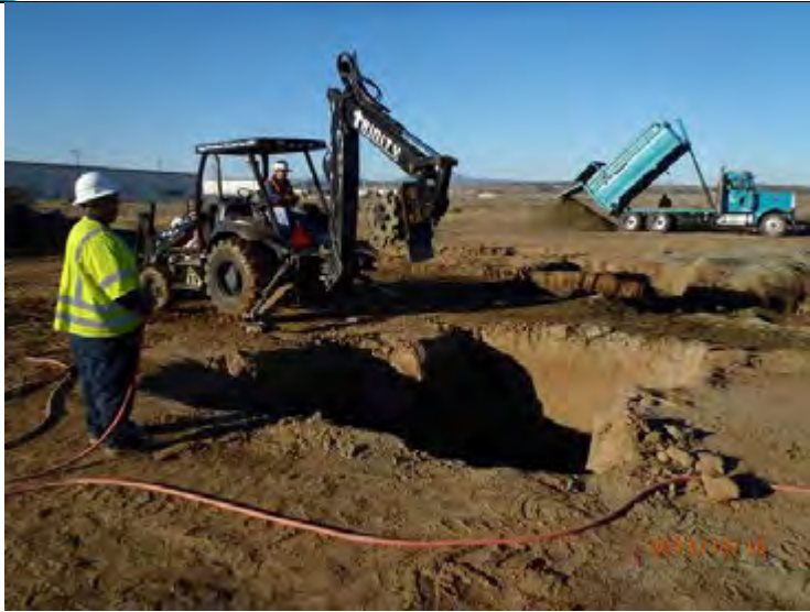
Importing soil, moisture conditioning and compacting 8" lifts to >90%
