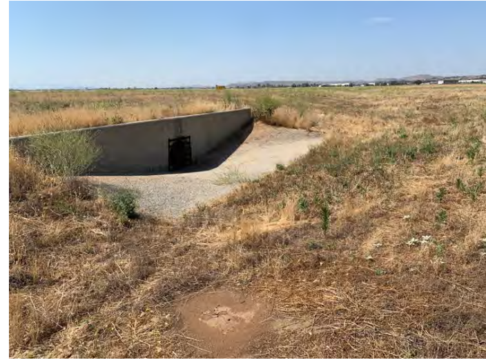
Photo 26. Overview of S-1. Photo taken facing south showing a culvert inlet (33.877202, -117.252005).
