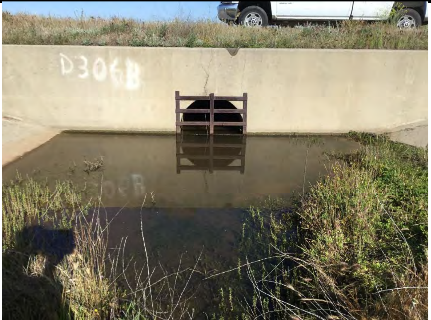
APRIL 2020 PHOTO LOOKING NW AT CULVERT OUTLET
