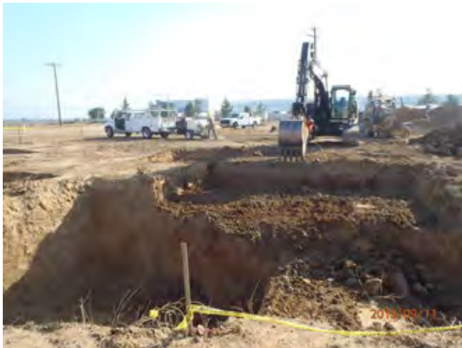
West side of excavation looking East from deep excavation area
