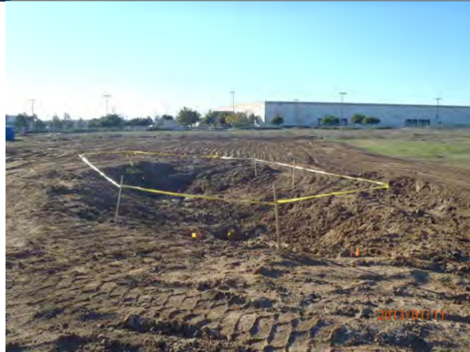
Looking south at the deeper excavation caution taped off
