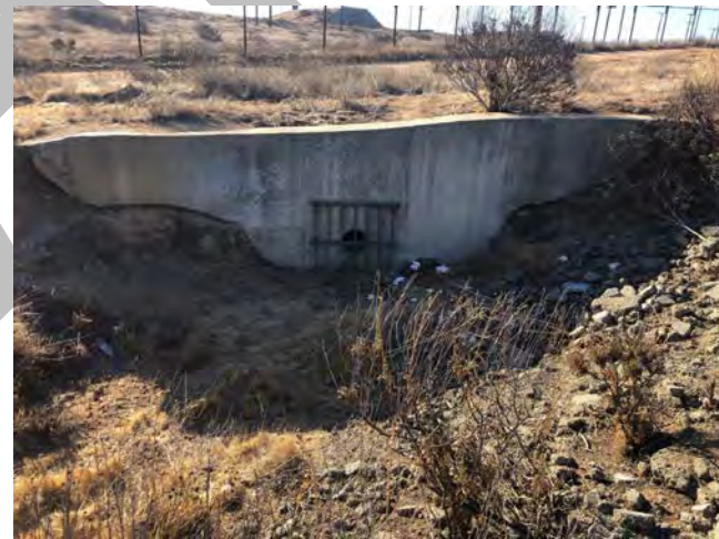
Photo 12. Upstream view of culvert that feeds into NWW-4, facing southeast (33.904782, -117.312060). August 6, 2021.
