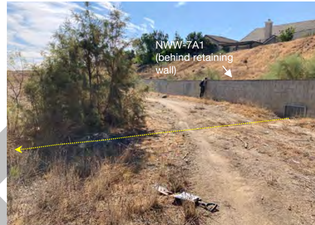
Photo 30. View of the upstream extent of NWW-7A (yellow dashed line), facing east, where flows from NWW-7A1 and NWW-7A2 travel through the culvert (33.898454, -117.313740). July 28, 2021.
