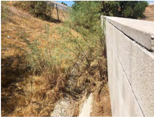
Photo 29. Downstream view of ODP 5, facing west, within NWW-7A1 (33.898451, -117.313362). August 6, 2021.
