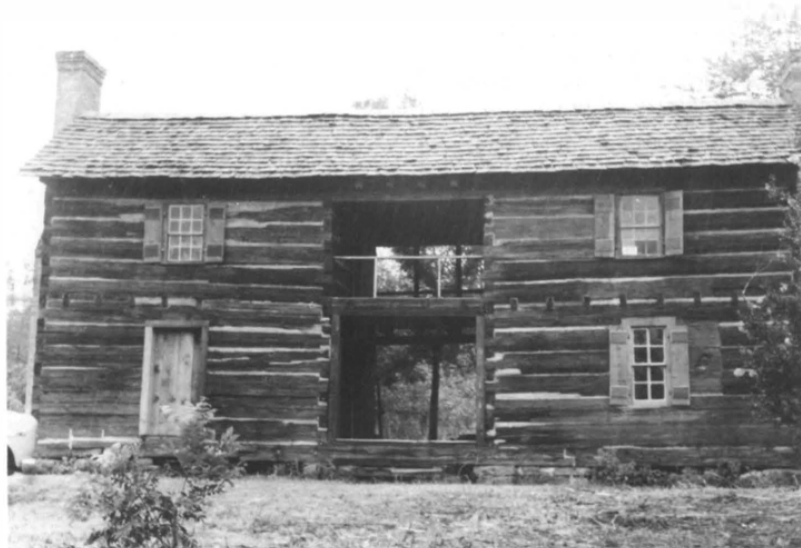
Looney House , Asheville vicinity, St. Clair County, Alabama. Examples of vernacular styles of architecture can qualify under Criterion C. Built ca. 1818, the Looney House is significant as possibly the State's oldest extant two-story dogtrot type of dwelling. The defining open center passage of the dogtrot was a regional building response to the southern climate. (Photo by Carolyn Scott).
