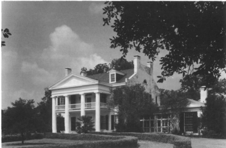
Richland Plantation, East Feliciana Parish, Louisiana. Properties can qualify under Criterion C as examples of high style architecture. Built in the 1830s, Richland is a fine example of a Federal style residence with a Greek Revival style portico. (Photo by Dave Gleason).
