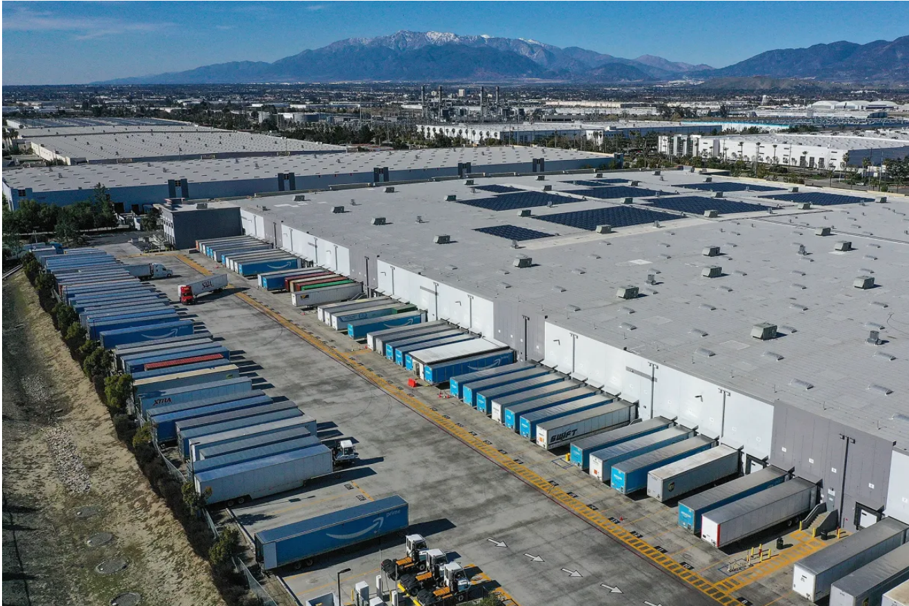
Large warehouses including an Amazon fulfillment center in San Bernardino on Jan 26, 2022. Photo by Jay Calderon/The Desert Sun
