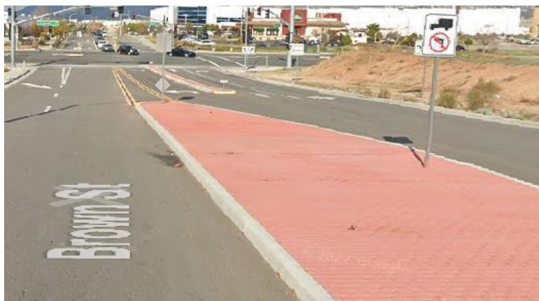
Figure A-7.1-2 Brown Street looking north towards Alessandro Blvd.
