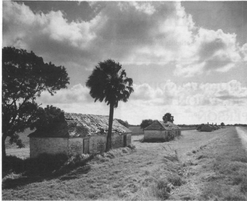
Criterion A - The Old Brulay Plantation, Brownsville vicinity, Cameron county, Texas. Historically significant for its association with the development of agriculture in southeast Texas, this complex of 10 brick buildings was constructed by George N. Brulay, a French immigrant who introduced commercial sugar production and irrigation to the Rio Grande Valley. (Photo by Texas Historical Commission).
