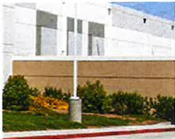
TILT-UP CONCRETE SCREEN
