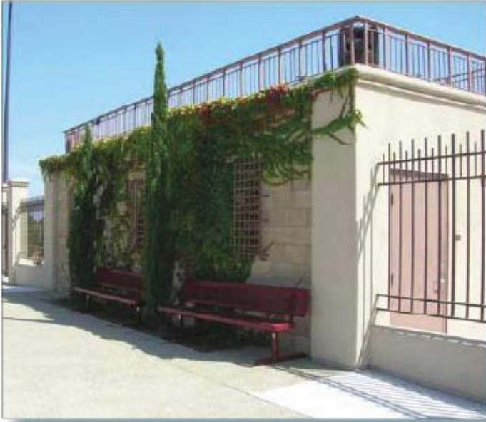
Mechanical room enclosure is complementary to the primary building design
