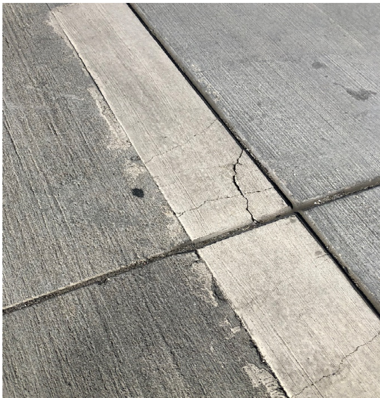
Photo 4: Small Patch (medium severity)
