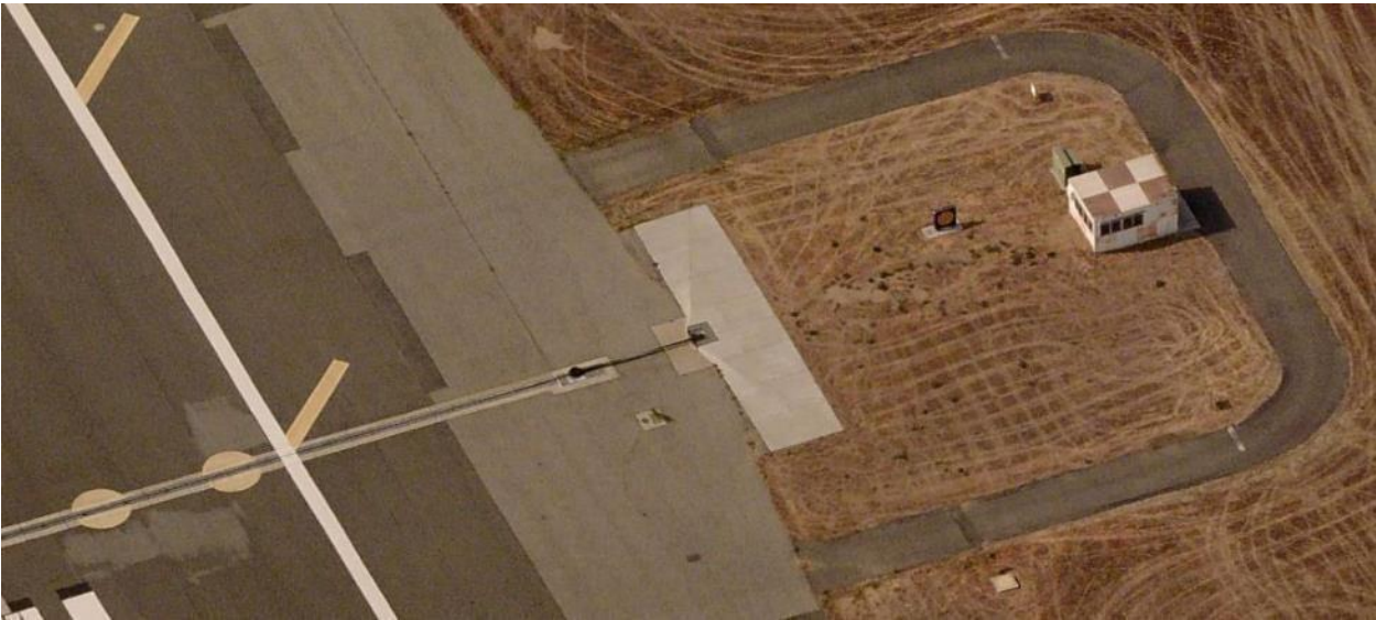
Figure 6.4 – BAK-12 Aircraft Arresting System and Associated Building
