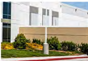
TILT-UP CONCRETE SCREEN WALL- 14' HIGH, MAXIMUM
