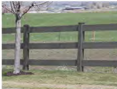
SPLIT-RAIL FENCING ALONG BARTON STREET MULTI-PURPOSE TRAIL & TRAILHEAD LOCATIONS- COMPOSITE, MATTE FINISH
